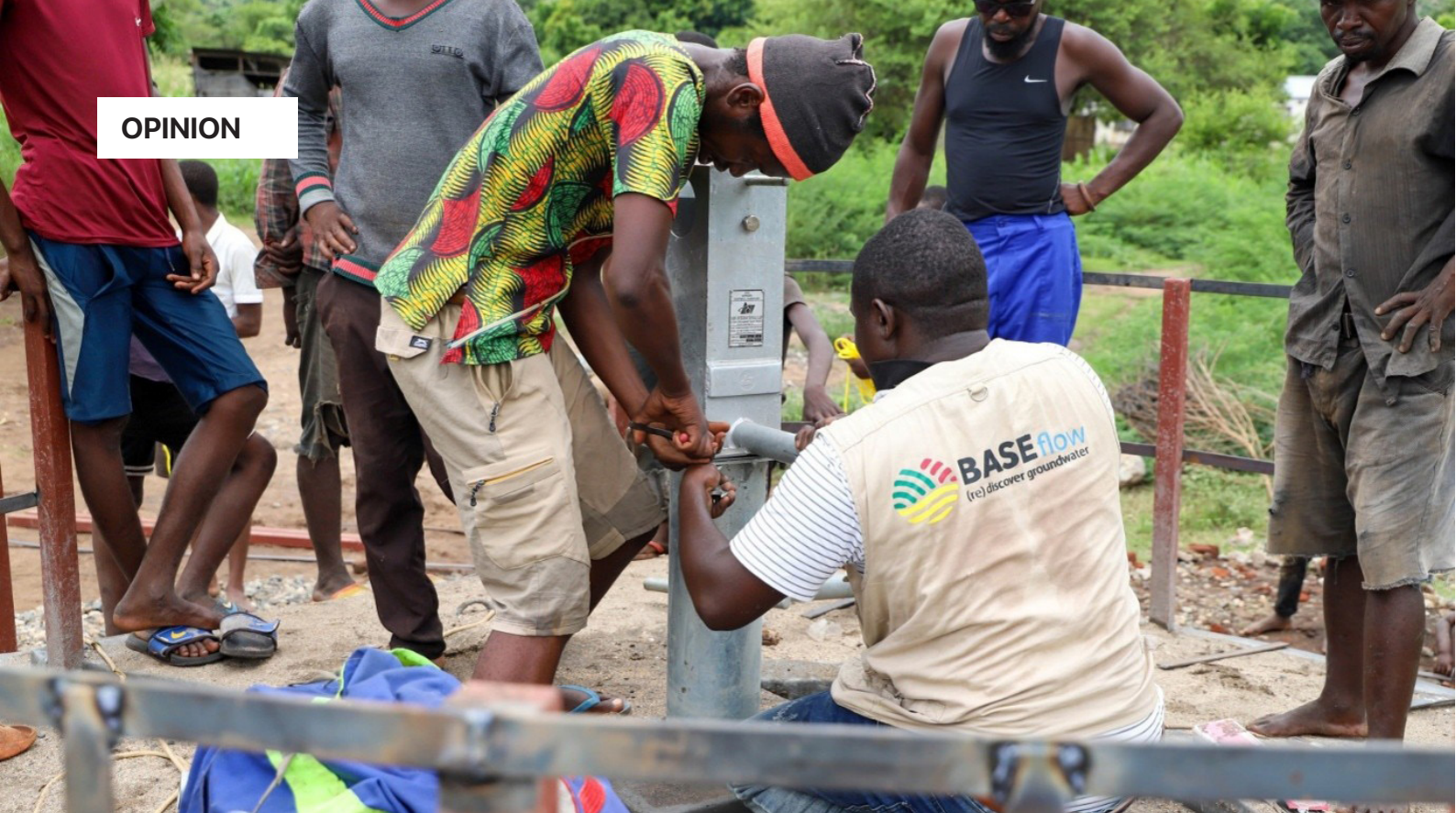
Maintenance works underway
