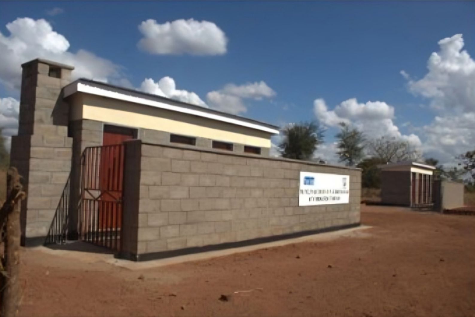
Two new latrine blocks
