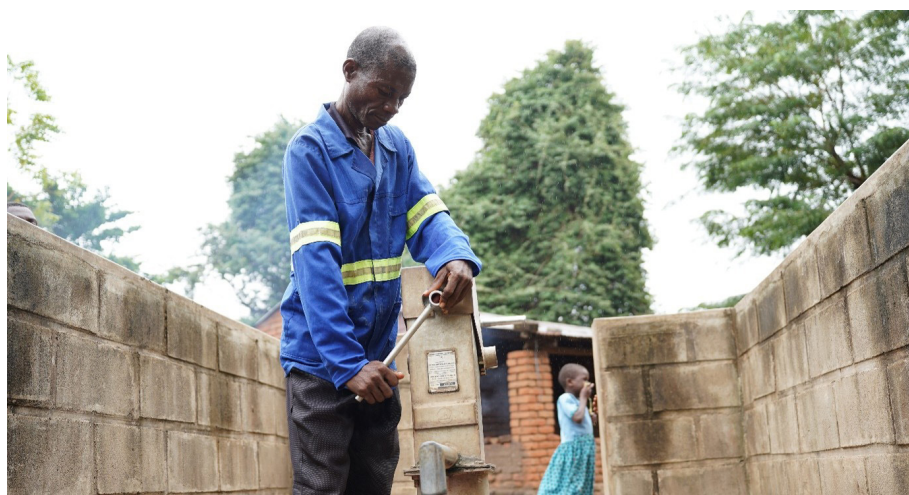
Area pump mechanic fixing a handpump (Chikwawa, Daniel Community)
