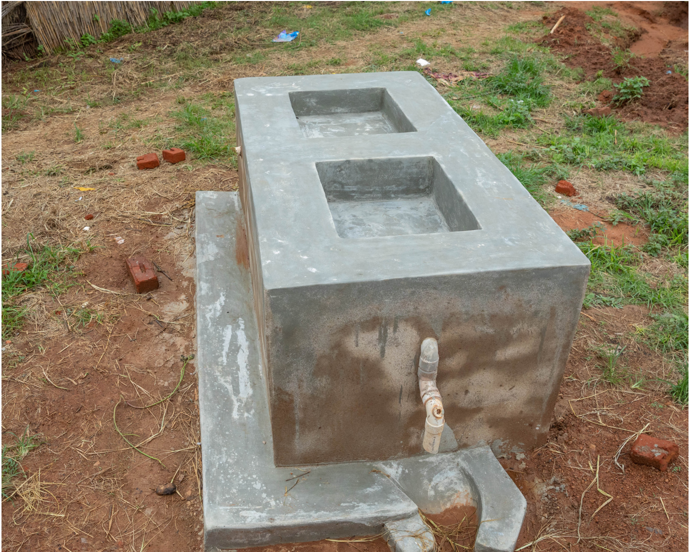
A newly constructed laundry station-Photo Credit WaterAid/Henry Ngulinga
