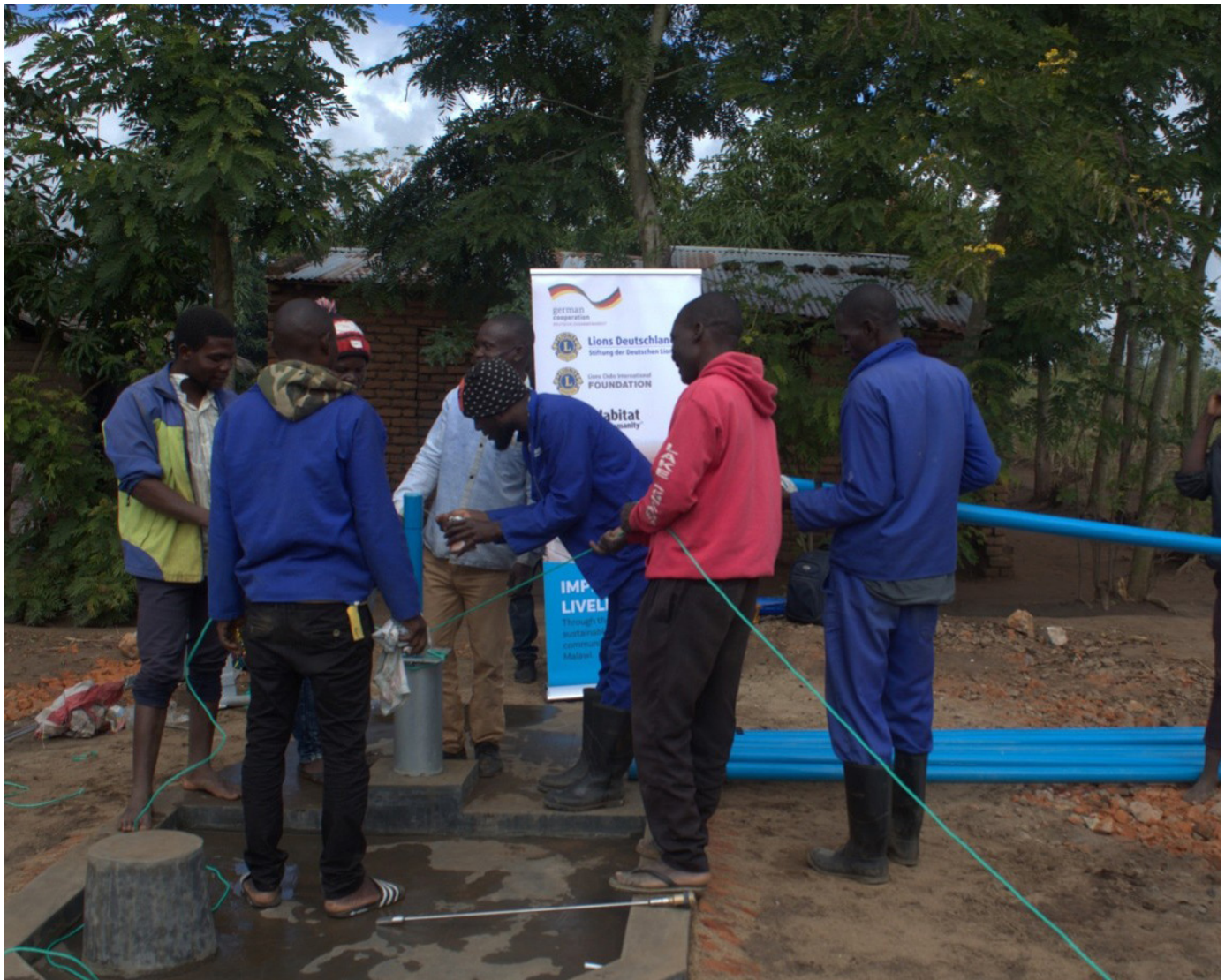
A team of trained Area Mechanics conducting pump installation at a rehabilitated borehole.
