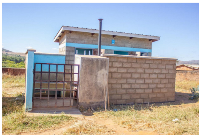
One of the newly constructed toilets
