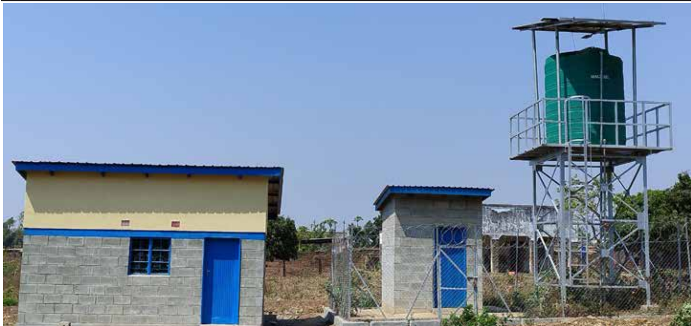
The solar system at Maravi Health Centre in Chiradzulo
