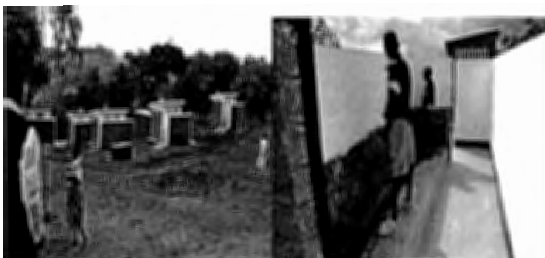
Examples of school sanitation facilities
