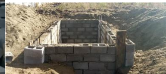
Completed flush latrine block Mchinji, pic 1, latrine block in progress Blantyre, pic 2 and septic tank for BT latrine block, pic 3
