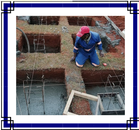
Construction of a 20 000L tank stand @Blantyre ETU, UNICEF
