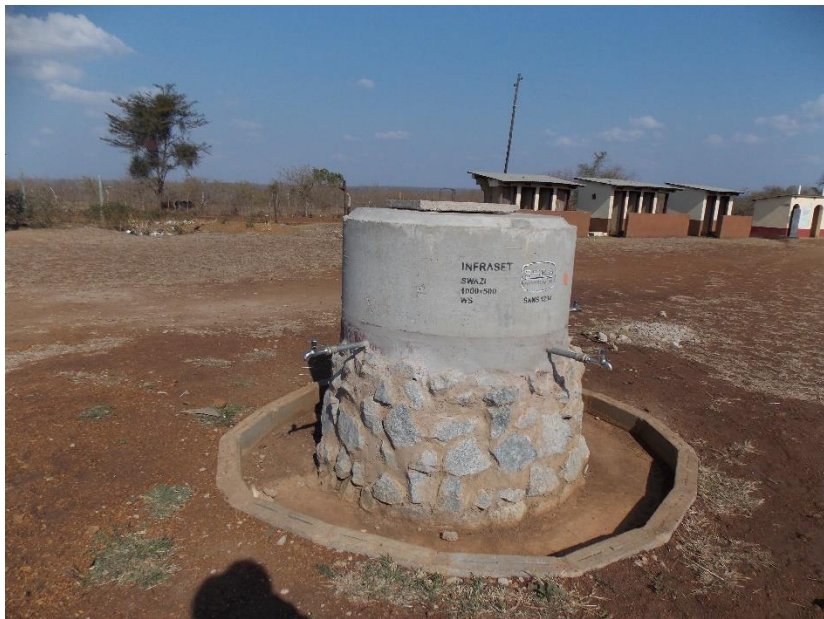
Figure 4 the hand washing facility that has been without water for several months
