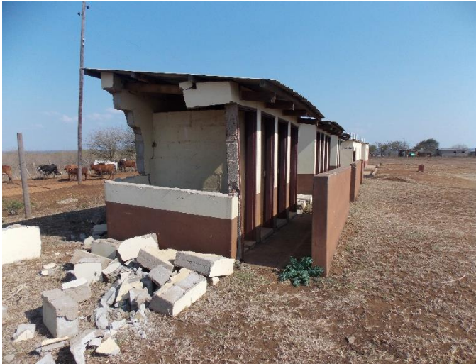
Figure 1 one of the girl's old toilets blocks
